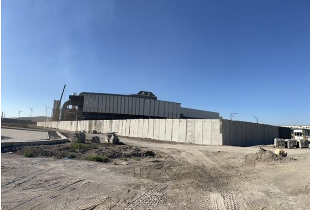
Photo-14: Border Walls of the Facility
