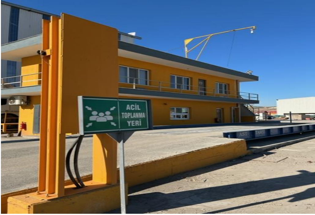
Photo-5: One of the Emergency Assembly Point Sign
