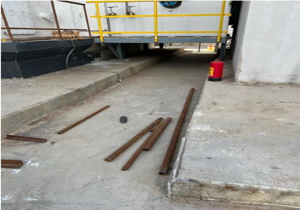
Photo-6: Unproper Material Storage
