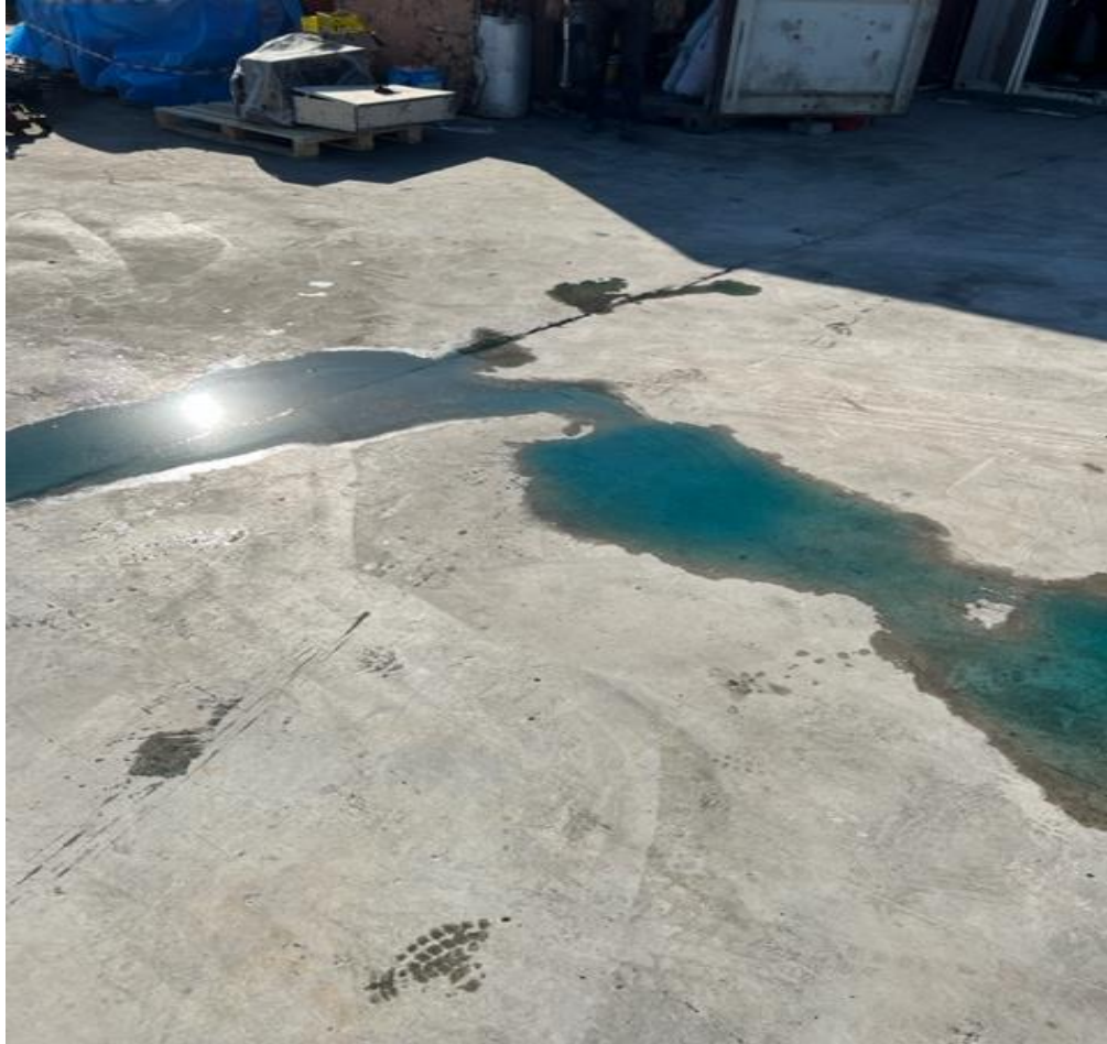
Photo-12: Chemical Accumulation on the Waste Storage and Maintenance Area
